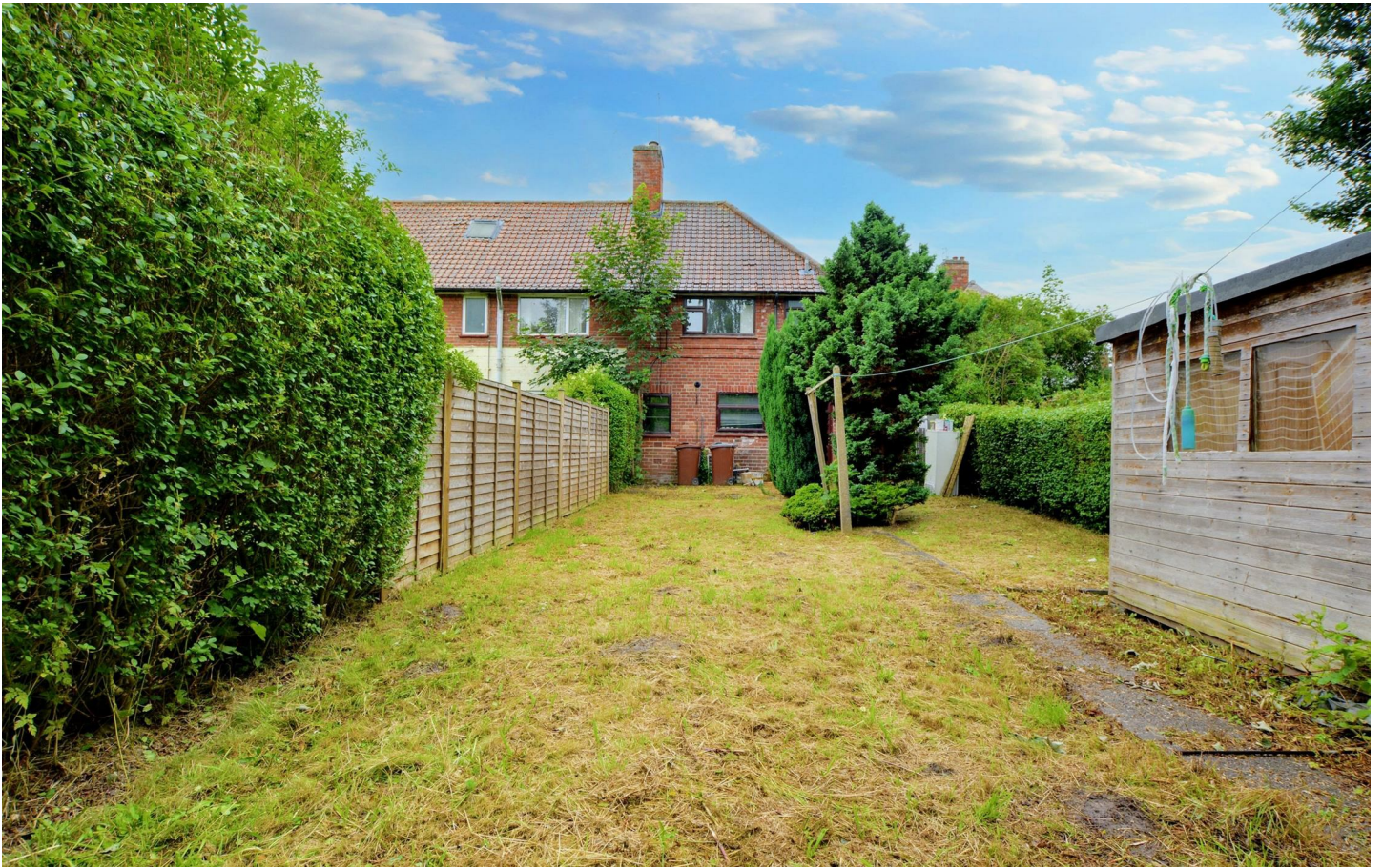
A Traditional Style Two Bedroom End Terrace House.
